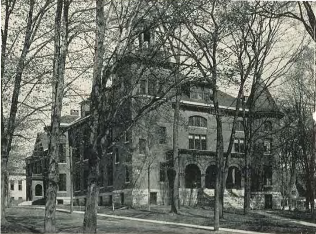
Administration Offices and Classrooms are located in the Main Building.
