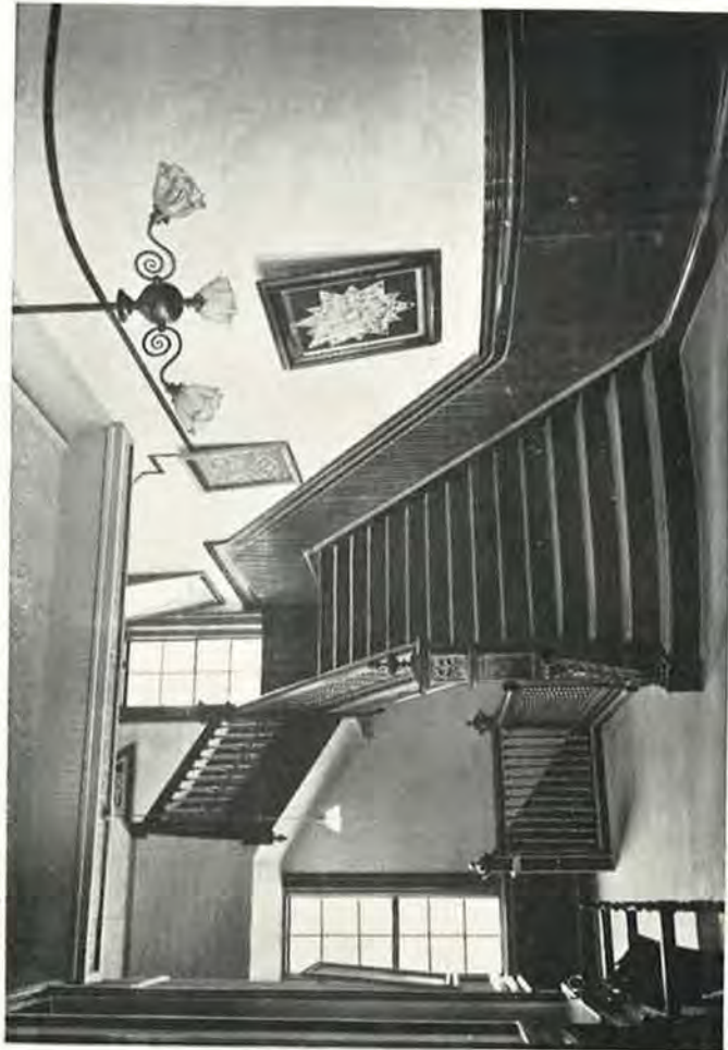
FARMINGTON STATE NORMAL SCHOOL.—MAIN STAIRWAY.
